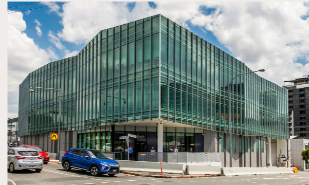
45 Commercial Road, Newstead
